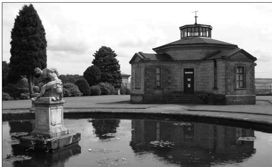
Fig. 5a 'Plan of the piers for Transit Circle' an undated drawing showing the dimensions of the stone piers for the transit circle by 'Mr. Jones' according to the note on the left edge with the initials JJS. b The building as it appears today.
